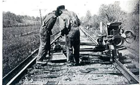
One machine is sufficient on this branch line rail laying job.
