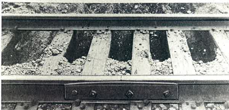
Crib cleaned to center of tie.
