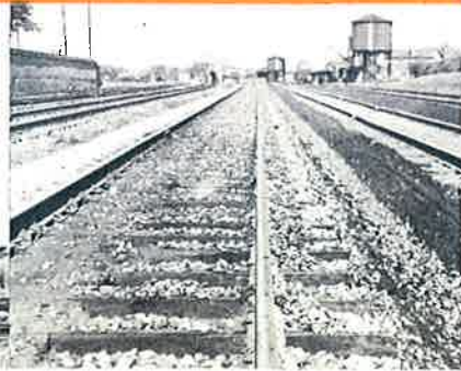
Intertrack and half-cribs cleaned and returned to track.
