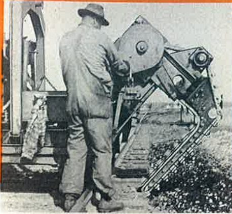
Boom raised ready to start digging.
