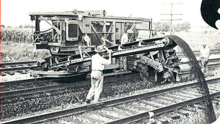
BALLASTEX-SCREENEX cleaning stone ballast
