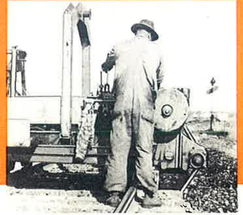
Digging completed to tie center.
