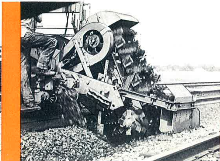
Rear view of Digging Boom. Note the cleaned ballast being returned.
