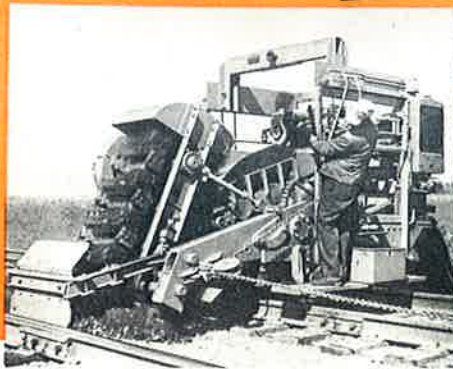
Wasting intertrack ballast.
