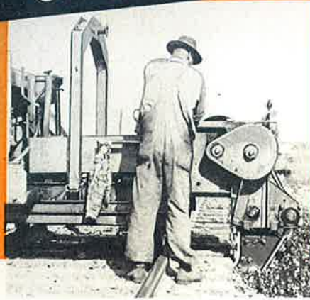
Boom under rail and entering crib.
