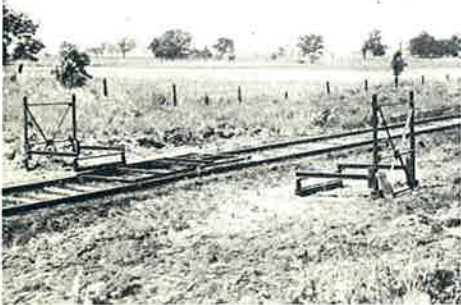
Cribex setoff in single track. Turntable placed in track.
