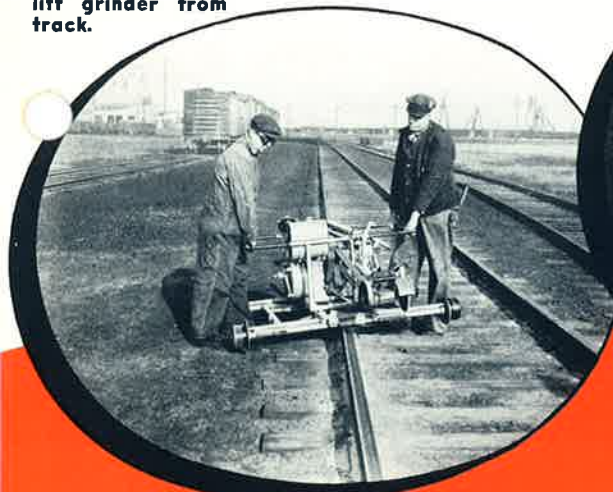
Swinging the arm to grind on oppo- site rail.
