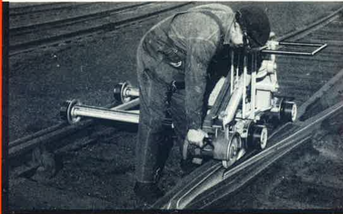
Grinding flangeways at frogs and crossings.
