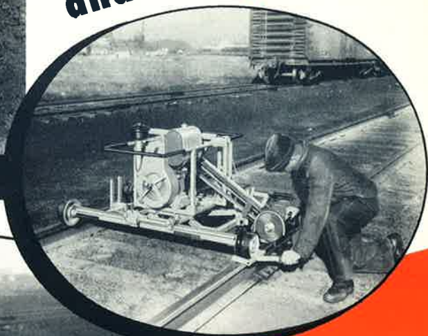
Slotting rail ends.
