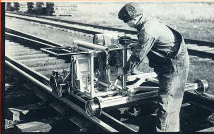
Adjustable spring tension maintains uniform pressure of wheel against stock rail or switchpoint.
