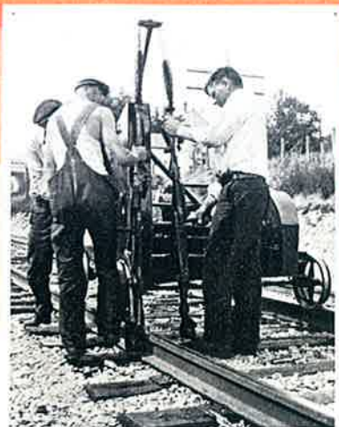
Here the machine pulled as many spikes as 12 men did by hand.
