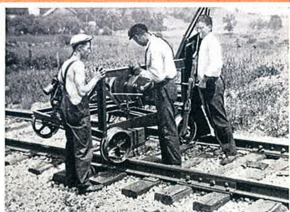
Turning the machine to pull on opposite rail.
