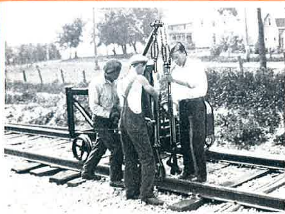
A single line relaying job under traffic.
