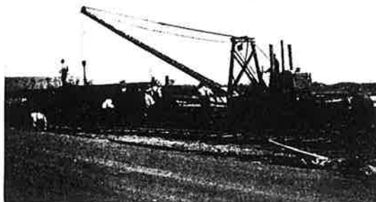
In moving up, the machine has a sufficient power to push the car of rails ahead for each setting.
