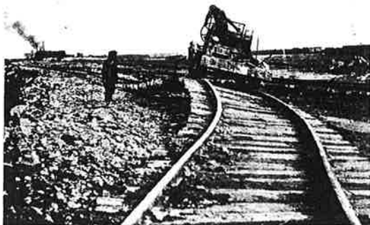
Shifting track in the construction of a railroad yard. With the Track Machine, it is not difficult to shift track to the inside of a curve.
