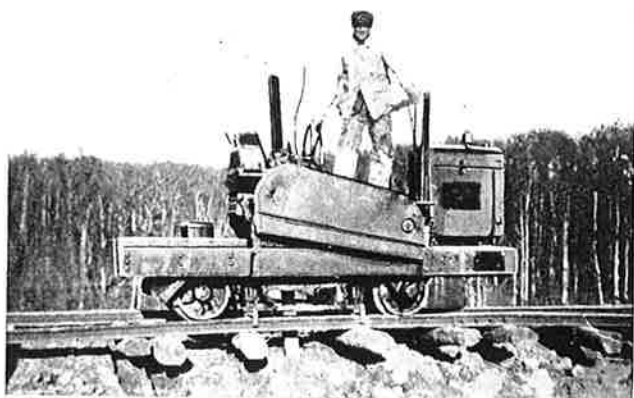
Another quarry shifting job; an easy task for the Track Shifter.
